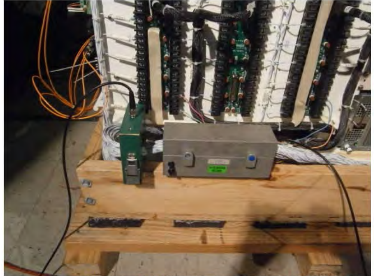
General Test Setup for CS115 Impulse Excitation on Signal Bundle 1
